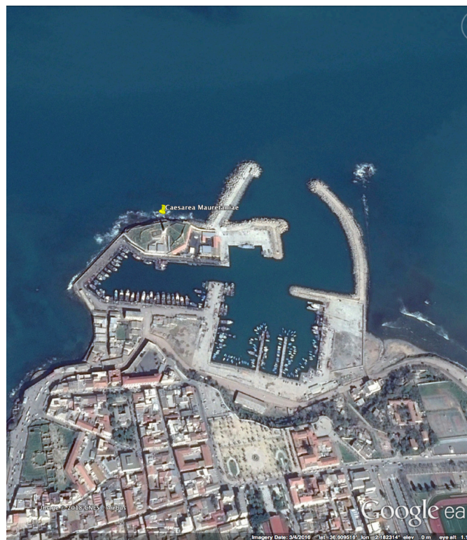
Fig. 6-29: The harbour at Cherchell in Algeria that was originally called Caesarea Mauretaniae and the site of a Roman lighthouse. It was situated on an island on the left of the image above, as indicated. 77
