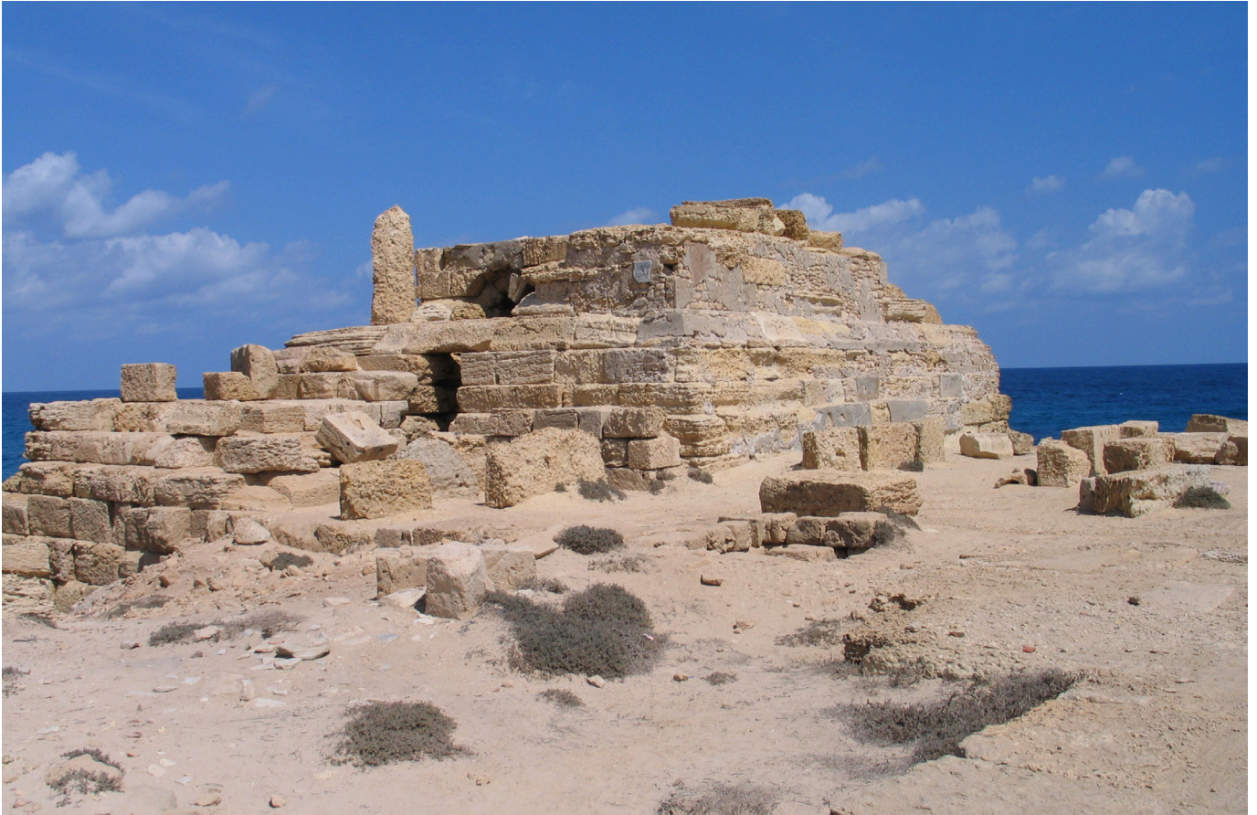
Fig. 6-35 (above): The remains of a large lighthouse originally constructed on the end of a mole at Leptis Magna in present-day Libya, 130 km east of Tripoli. The square base is clearly visible, and what appear to be steps on the left. The sea is continually attacking the foundations and badly affecting the remains on the seaward side. 83 Fig. 6-36 (below): Satellite image of Leptis Magna and the old harbour now completely silted up. The red line indicates the original edges. 84
