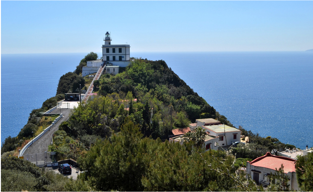
Fig. 6-20: The present lighthouse (E1620) at Capo Miseno (Cape Misenum) viewed from the north. 61
