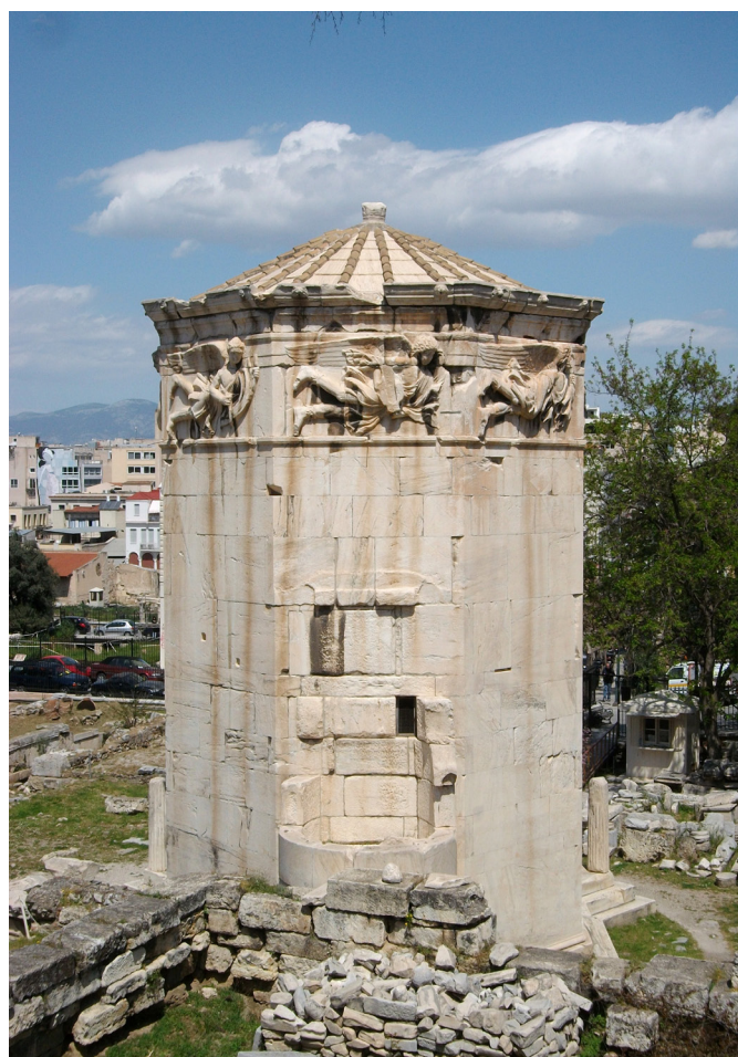
Fig. 2-16: The Torre Dels Vents in Athens is a well-preserved tower and a strong indicator that the shape of the central octagonal section of the Pharos of Alexandria was chosen because of its relationships to the eight winds of the compass rose, so essential to mariners of ancient times. 72
